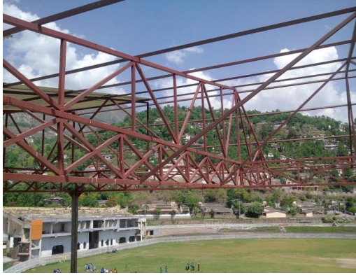
CGI Roofing with Steel Structure
