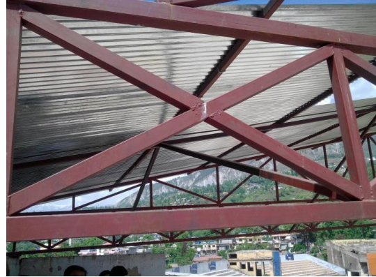
CGI Roofing with Steel Structure
