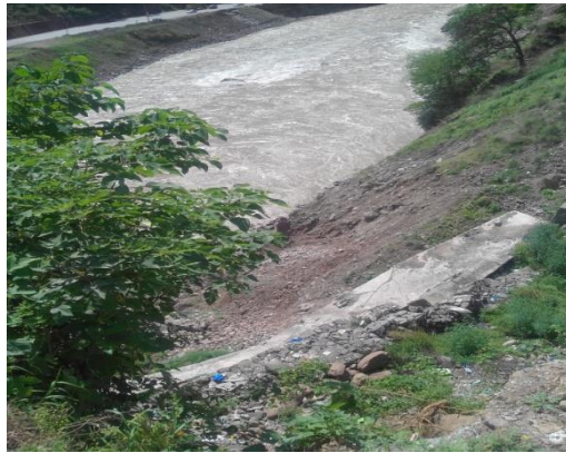
Protection work at disposal point being eroded
