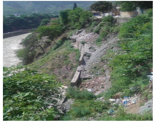
Protection work at disposal point being eroded
